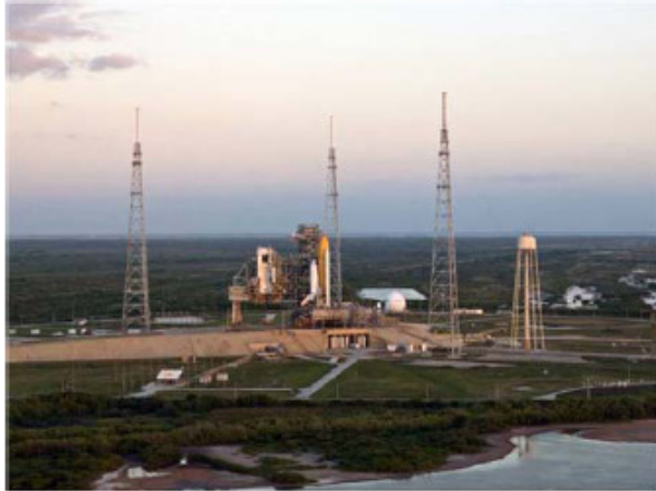
Figure 1. Lightning protection system of LC39B, Kennedy Space Center, Florida. Seen at the launch pad is the standby rescue Shuttle during the Hubble repair mission in 2009.
